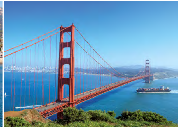
Golden Gate Bridge in San Francisco
